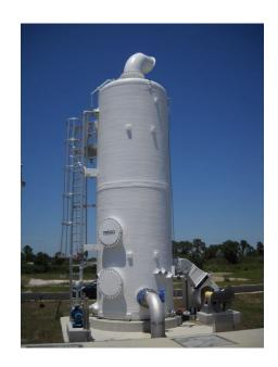
The pack tower air stripper was developed to remove toxic volatile contaminants from water. It is designed as a counter-current system where the air moves up and the water moves down the tower column and interacts with the packing media. The packing media provides a large surface area for mass transfer and stripping of the contaminants
